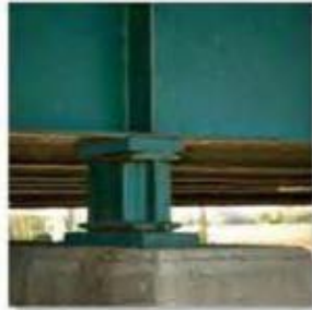
The rocker support for this bridge girder allows horizontal movement so the bridge is free to expand and contract due to a change in temperature. (5)
