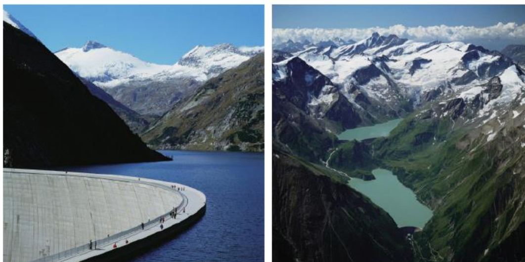
Figure 9.10 Storage power plants with reservoirs: Malta (left), Kaprun in Austria (right). Source: www.verbund.at .
