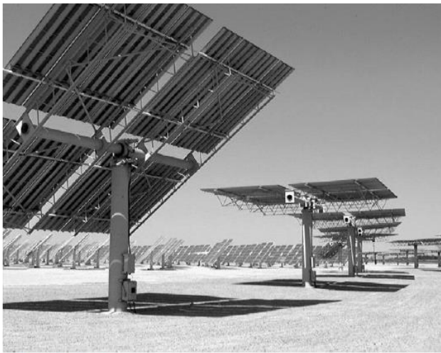
FIGURE 3.22 Detail of a heliostat.
