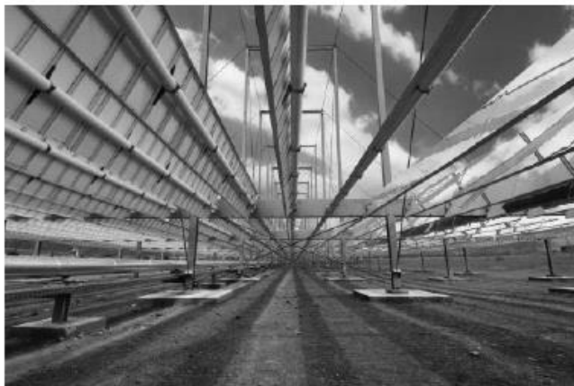
Figure 3.7 Here, one sees the support piping for the mirrors (Photo DLR).
